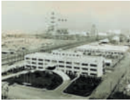
Office of Oita Petrochemical Complex
