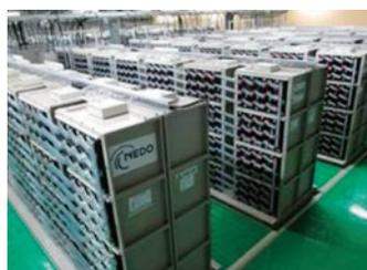
Figure 2 Advanced lead-acid battery systems which were installed on Izu-Oshima
